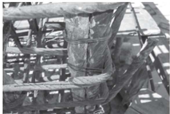
Figure 3. Insufficient hook length of ties in columns.
