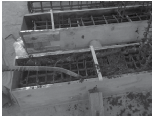
Figure 7. Placement of concrete in formwork with proper compaction through mechanical vibration.
