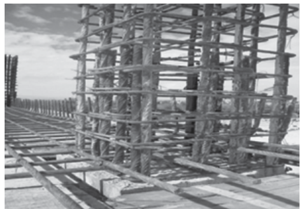
Figure 4. Improper location of lap-splices.
