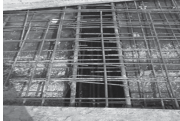
Figure 2. Staggered spacing of stirrups in beams.
