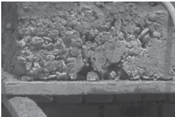
Figure 1. Honeycombed cast concrete.
